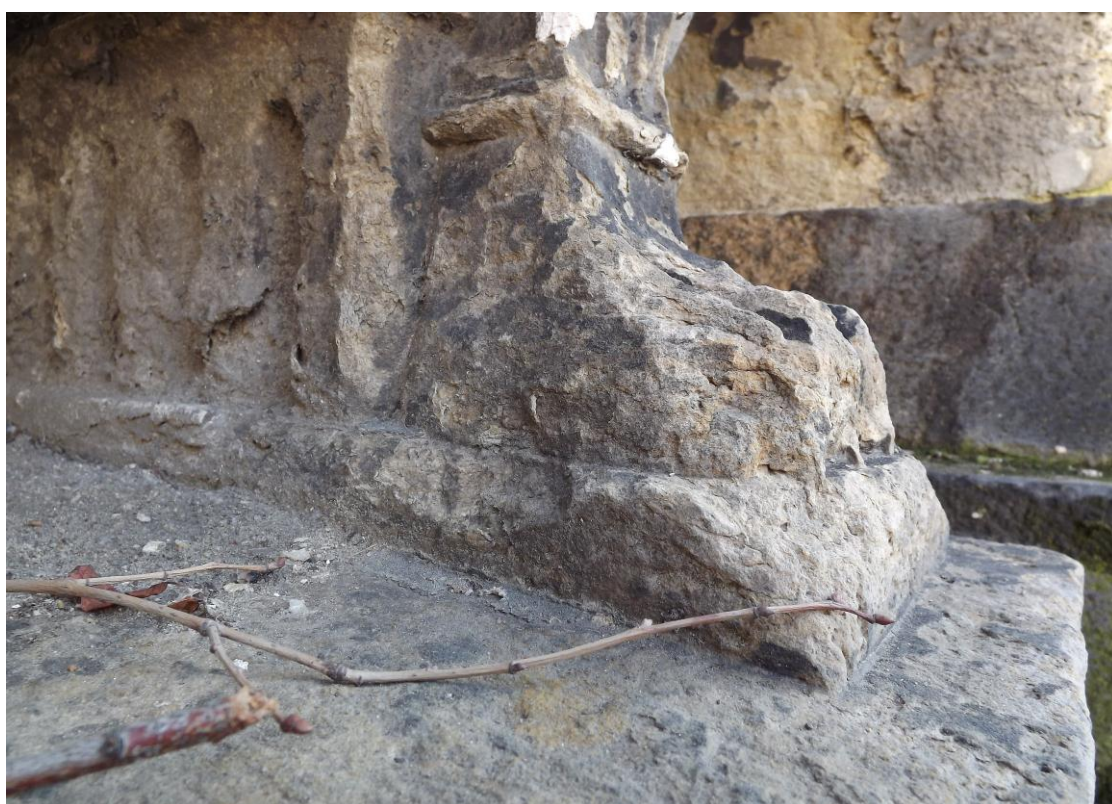
Detail degradace nohy
